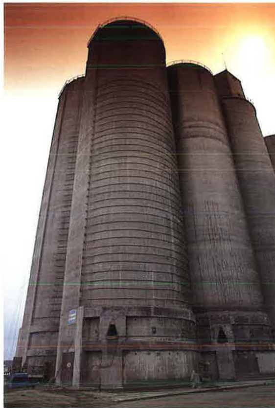
Reinforcement of grain silos in the port of Brest
