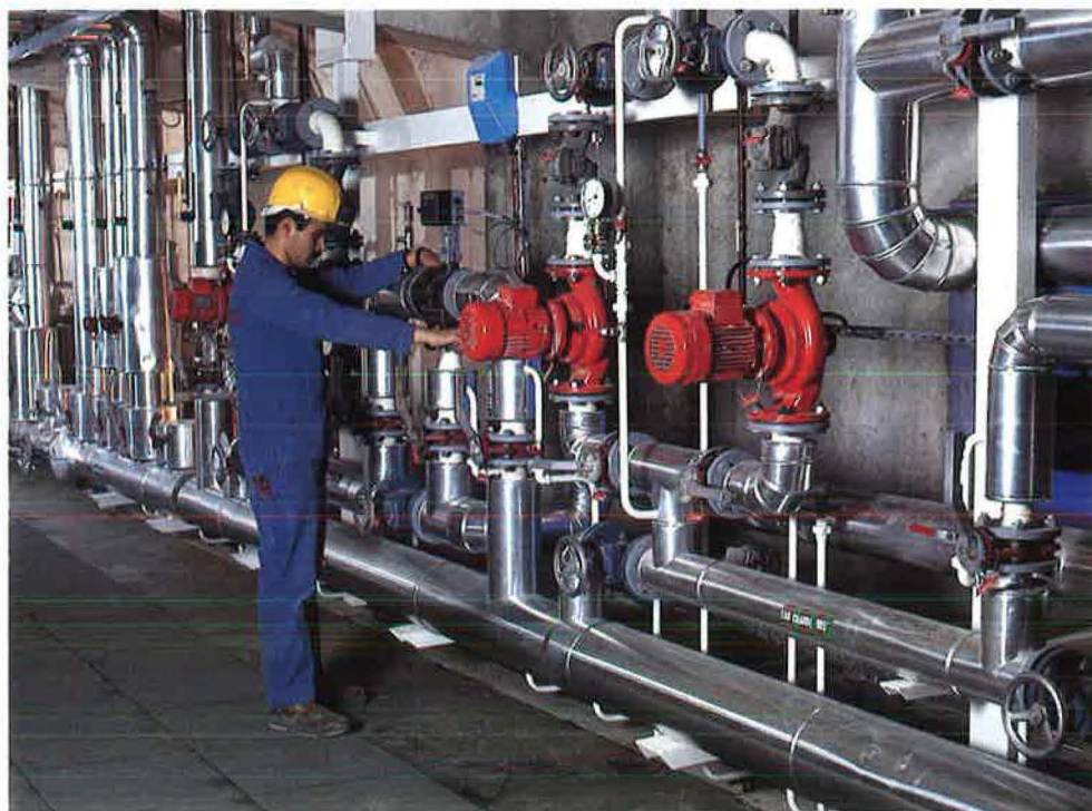
Air conditioning installation for Terminal C at Charles de Gaulle airport in Roissy
