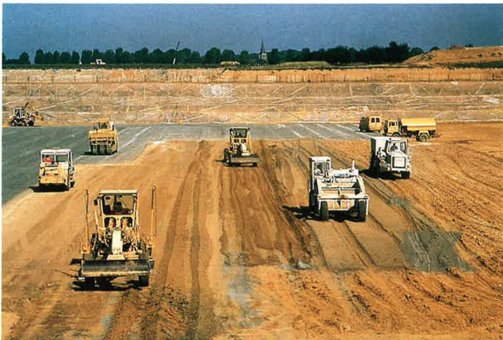
Construction of one of the platforms at the new Renault research centre in Guyancourt
