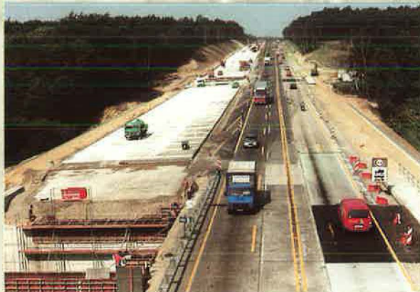
VBU: work on the A10 motorway near Berlin
