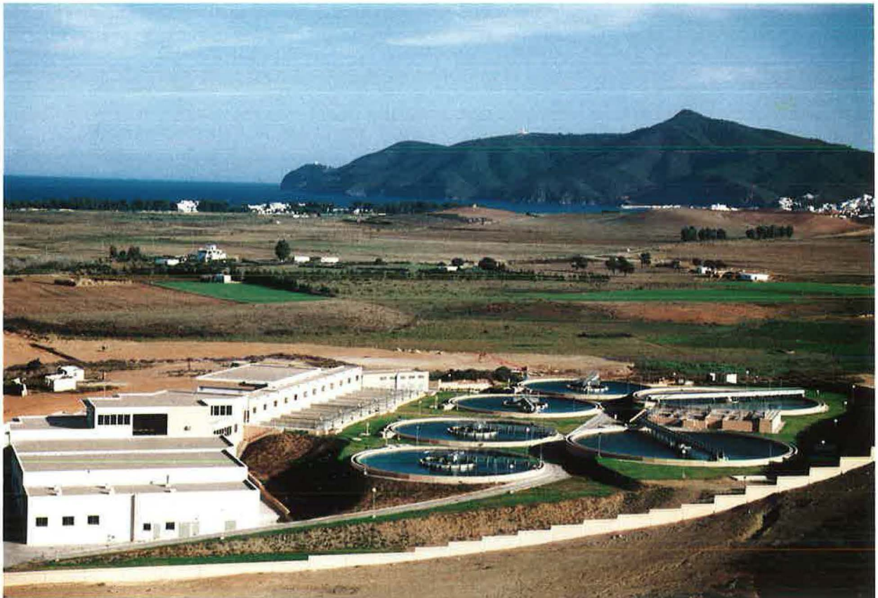
Drinking water treatment plant for the town of Tetouan, Morocco
