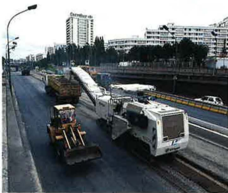
Resurfacing work on the Paris ring road
