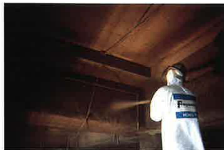
Electric corrosion protection of Kwai Chung Terminal 4, (Hong Kong)
