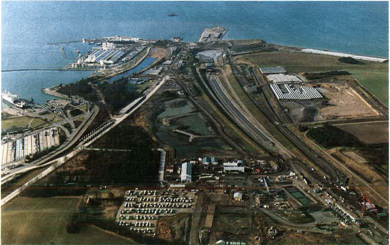
Aerial view of the site of the Storebaelt rail tunnel between the islands of Seeland and Sprogø in Denmark
