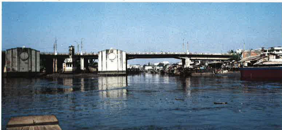
Reinforcement of bridge Y in Ho Chi Minh City, Vietnam
