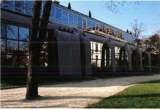
Sogea: renovation of the Victor Duruy secondary school in Paris
