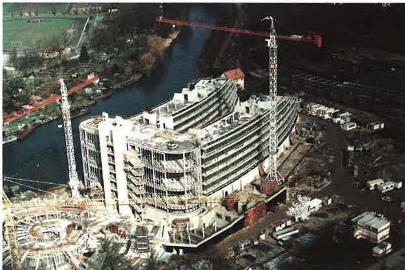
Construction of the Centre for Human Rights in Strasbourg by Urban, a subsidiary of Sogea
