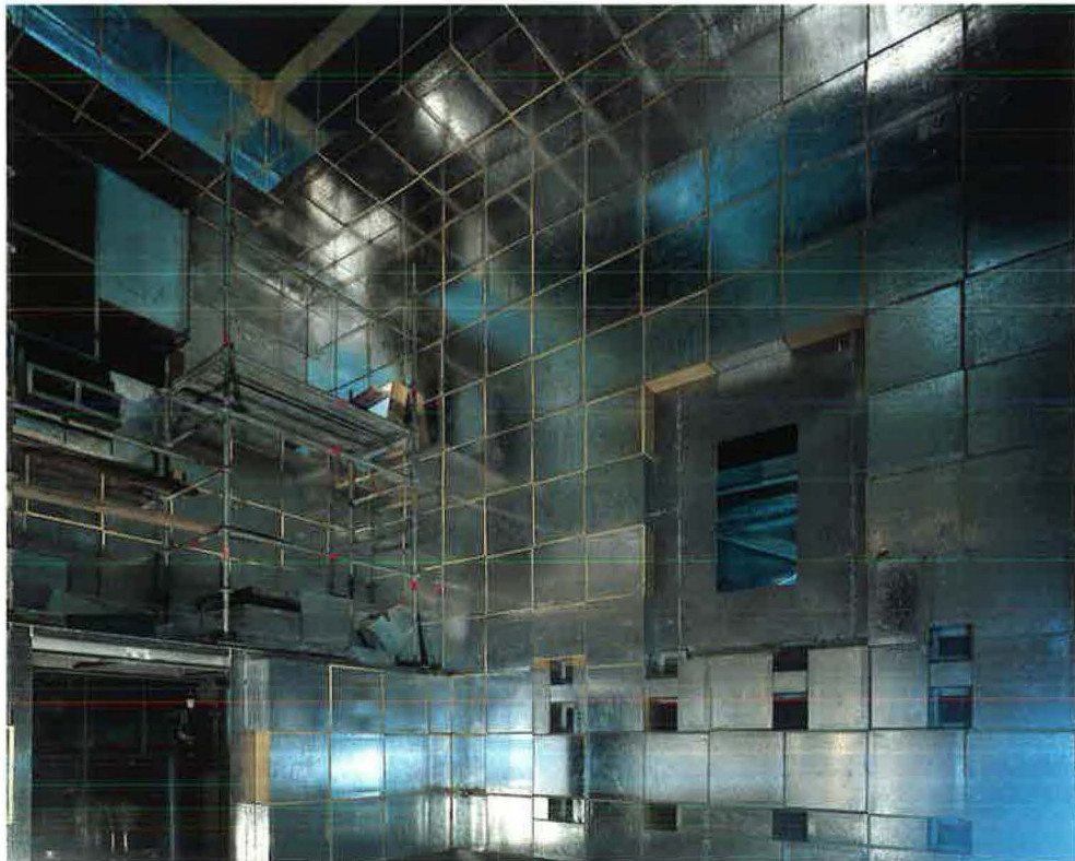
Thermal insulation of the European transonic wind tunnel (ETW) in Cologne (Germany)
