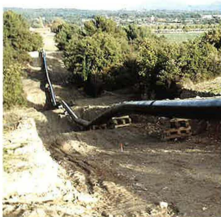
Section of the 70-km pipeline between the natural gas storage facility in Manosque and Cabriès in the Alpes-de-Haute-Provence
