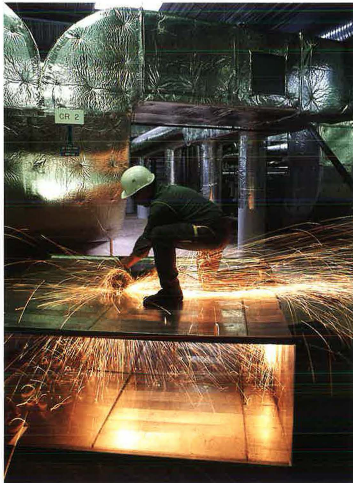
Air conditioning work for the Philips Composants plant in Dreux
