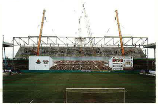
Norwest Holst: construction of the new Arsenal football stadium near London
