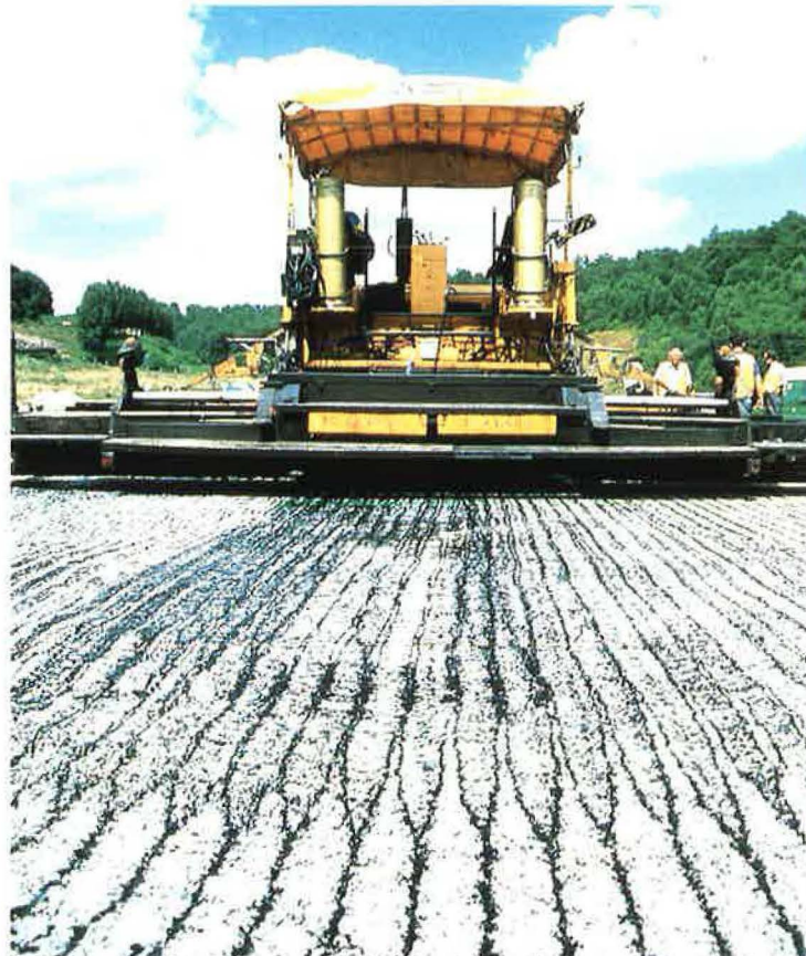
Work on the roadway of the new bypass northeast of Rouen
