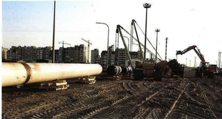
Denys laying a section of pipeline in Zeebrugge, Belgium to transport natural gas from Norway
