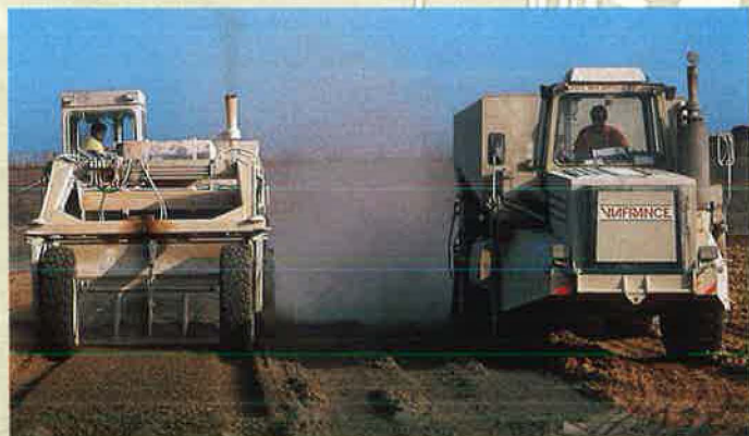
Viafrance : roadway improvement work in Guyancourt (Yvelines)
