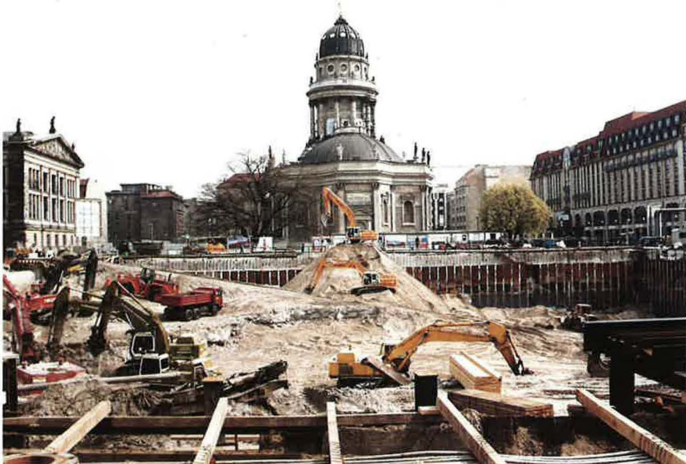
Foundations for the future Friedrichstadt Passagen building complex in Berlin
