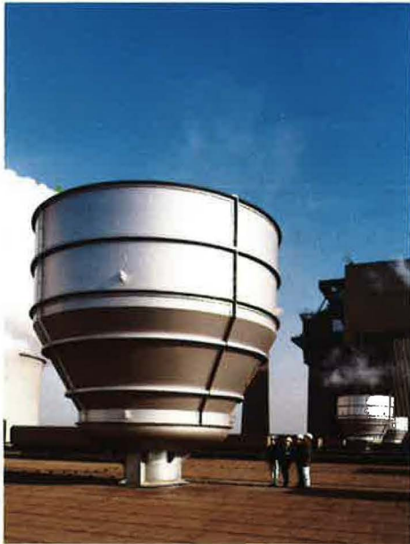
Silencers installed in the Niederaussem power station near Cologne
