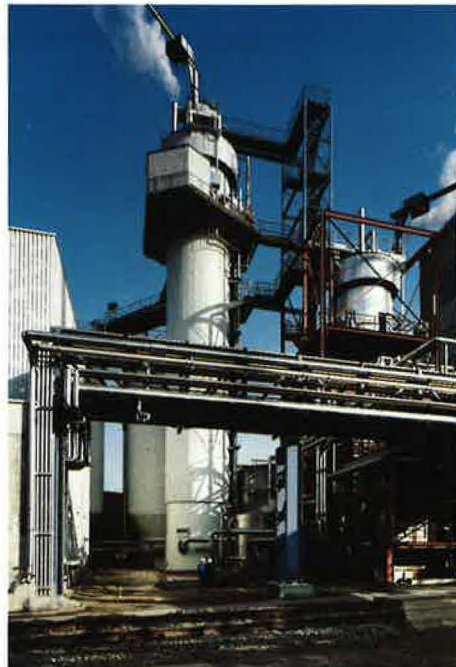
Thermal insulation work performed for Bayerische Zellstoff in Kehlheim
