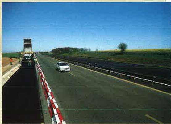
Cofiroute : widening the A11 motorway to six lanes between Chartres and Paris
