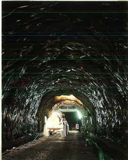
Campeon Bernard SGE: drilling of the Puymorens tunnel in the Pyrenees
