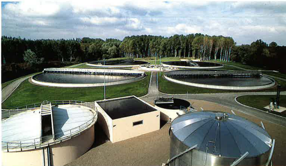
Barberey sewage treatment plant in Troyes, constructed and operated by Sogea
