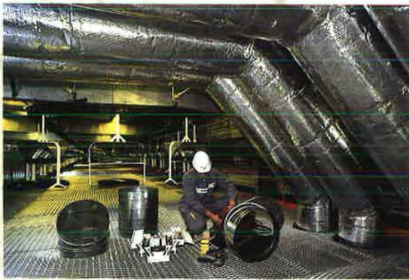
Tunzini : air conditioning work for Philips Composants in Dreux
