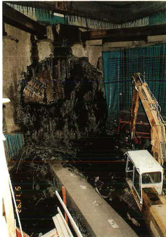
Drilling for line 2 of the Lille-Roubaix metro
