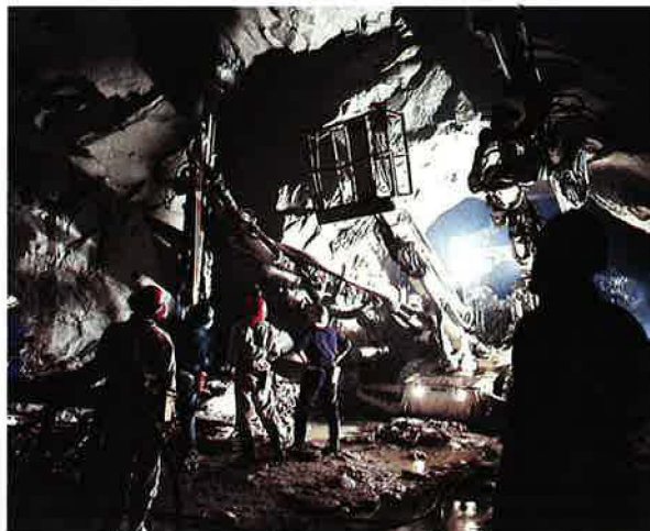
Drilling of a water supply tunnel in Lesotho : 20 km drilled in 1992, out of a total of 65 km
