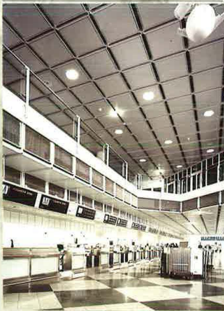
G + H Montage: interior work on the new Munich airport
