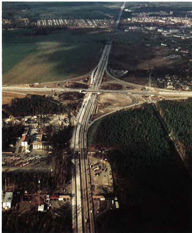
Roadwork performed by VBU on the Hermsdorf motorway interchange south of Leipzig
