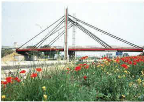
Upper level of the A6 motorway in Beaune
