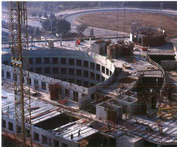
Construction of the new SGE Group head office in Rueil-Malmaison.
