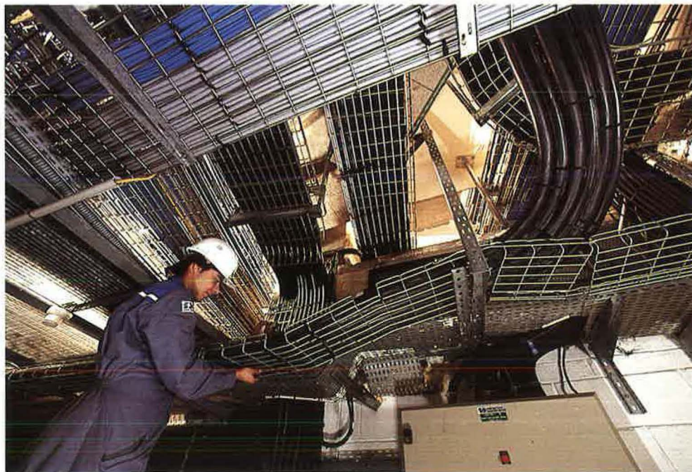
Installation of data network cabling for a Paris branch office of Société Générale
