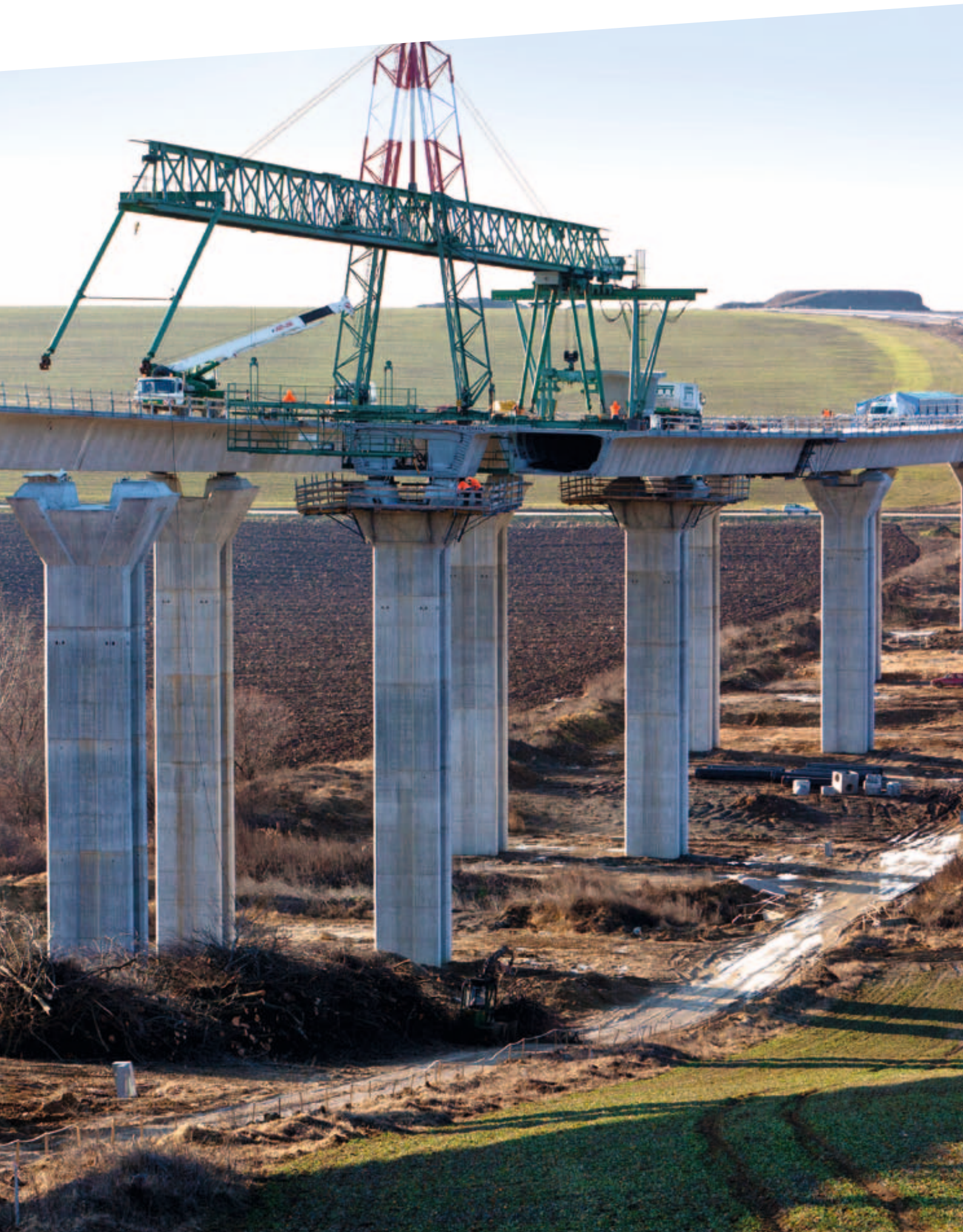
Worksite of the R1 expressway in Slovakia.
