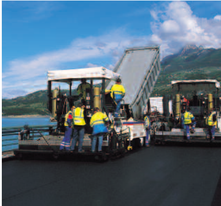
RENOVATION OF THE SAVINES BRIDGE (FRANCE)
