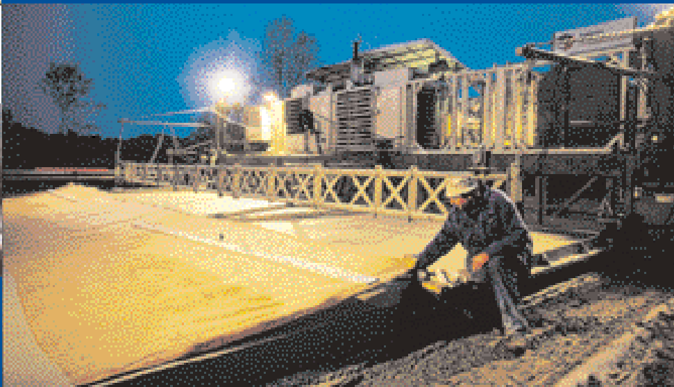
^ Rehabilitation of the concrete pavement of a 2 x 2 lane road in Hannover, Germany.
