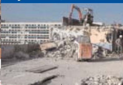
✓ Demolition of the Gérard-Philippe housing project building in Gennevilliers using a high-reach shovel, France.
