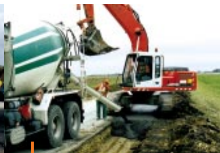
3 - France Widening of the RD17 highway at Ouarville (Eure et Loire) using the Scorcan product, a self-compacting bottom-ash concrete.
