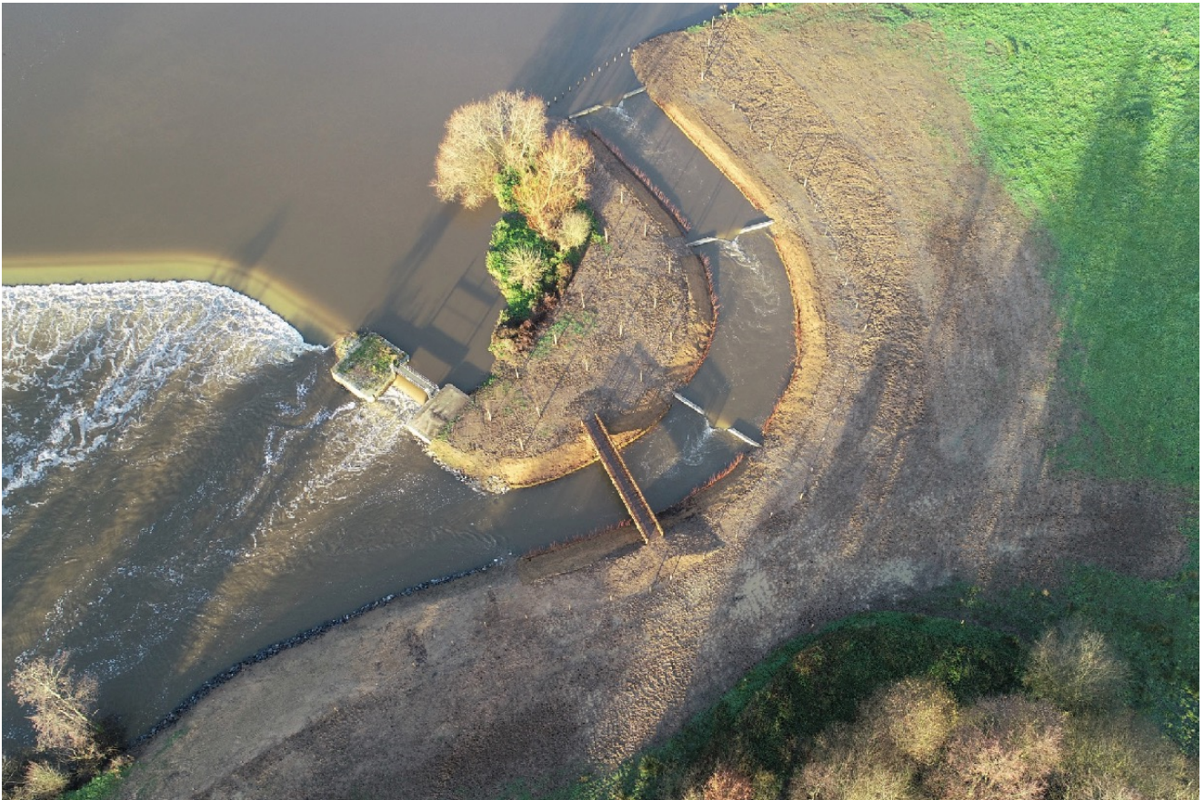
Restoring hydraulic continuity by building a fish pass on the river near La Jaille-Yvon (western France) enabling various fish species to swim upstream.
