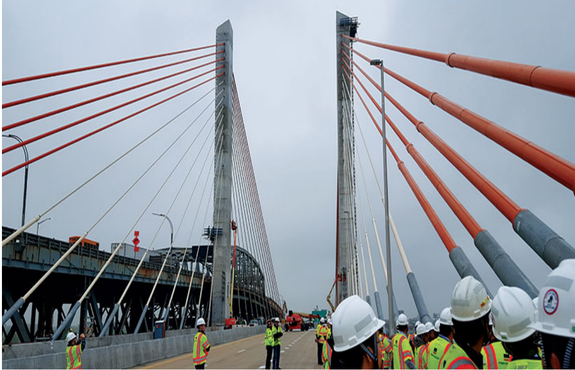
VINCI Construction (Freyssinet) cables for the new Kosciuszko Bridge in New York City
