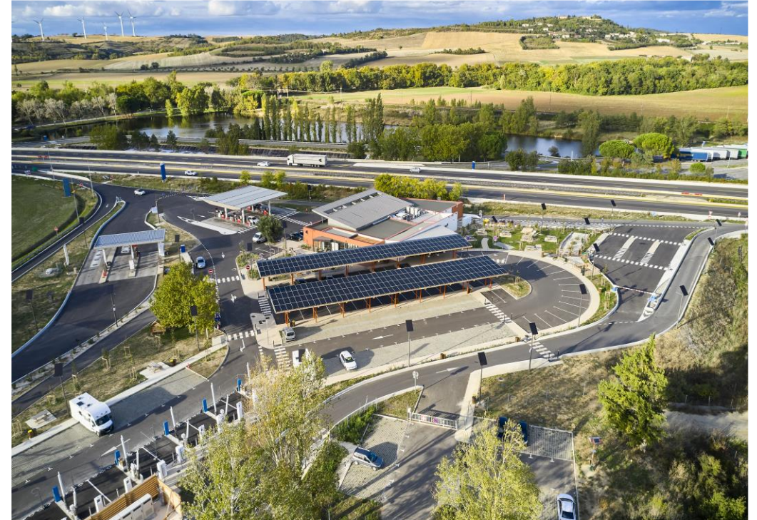
Shadehouse with photovoltaic panels installed on the Port Lauragais service station of the A61 motorway (Toulouse area)
