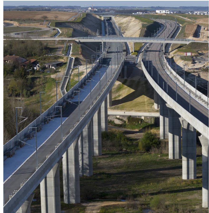
Tours-Bordeaux HSL: Auxance viaducts
