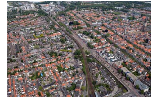
Rail tunnel in Delft (CFE)
