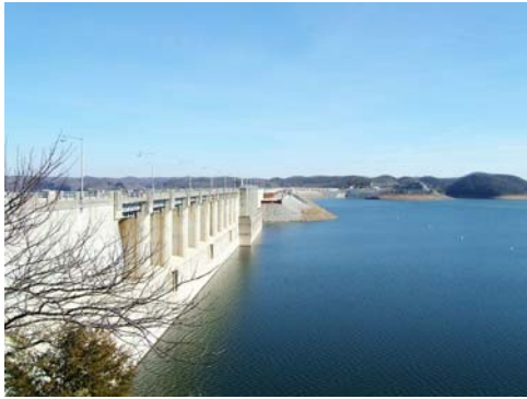
Dam in the United States (Solétanche)
