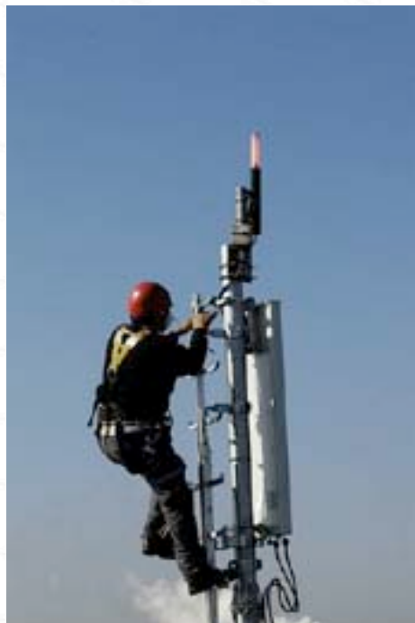
Installation of radio sites for SFR
