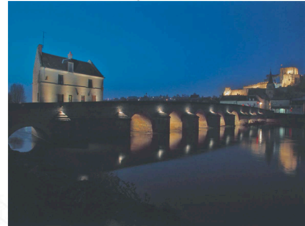
Heritage enhancement (XI th century Montrichard bridge – Loir et Cher)
