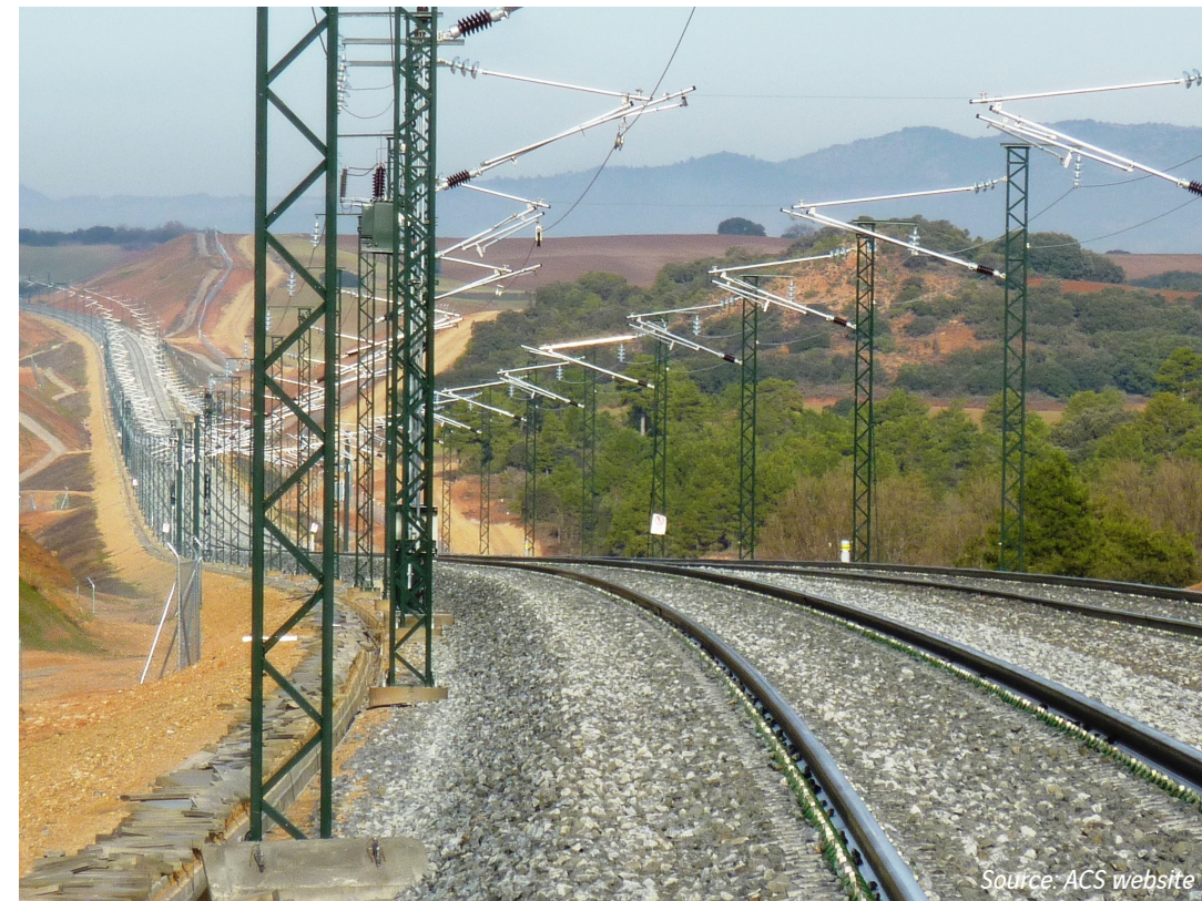
Installation of overhead contact lines on the high-speed rail line between Madrid and Valencia (Spain)
