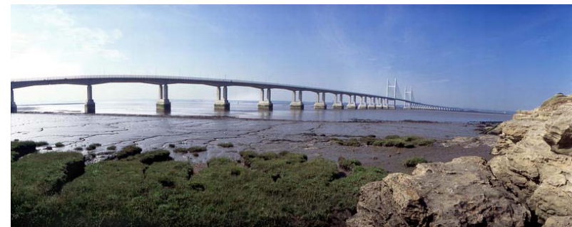
Severn Bridge (United Kingdom)
