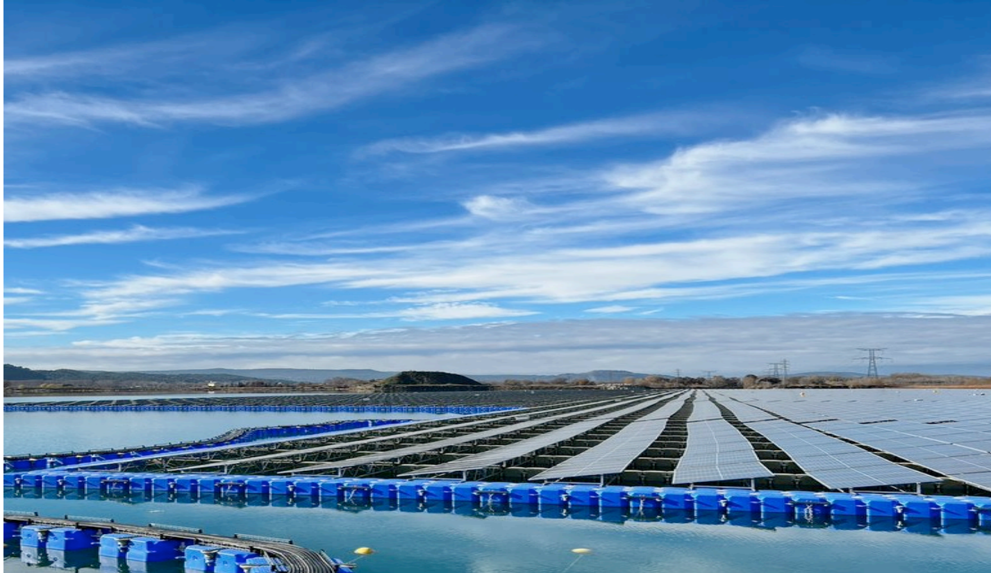
Construction of a 15 MW floating solar PV plant in Peyrolles-en-Provence (France)
