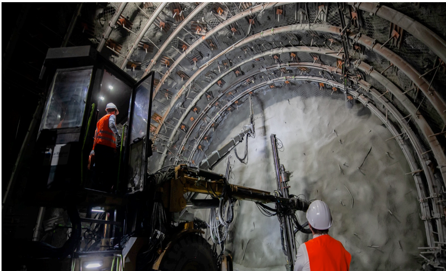
Works in relation to the Lyon-Turin rail link project
