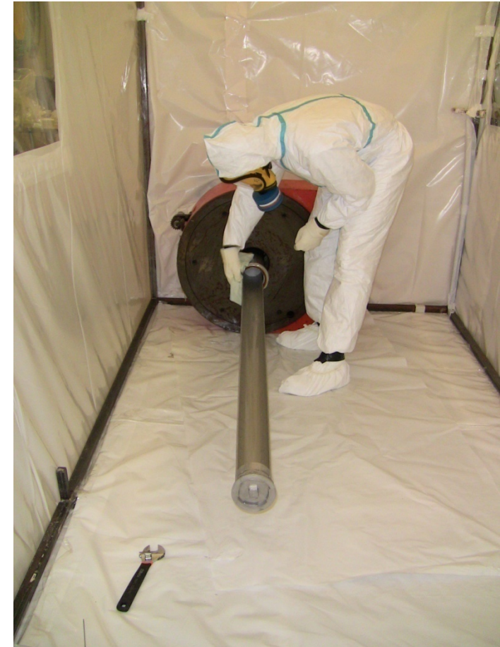
Decontamination, La Hague, France
