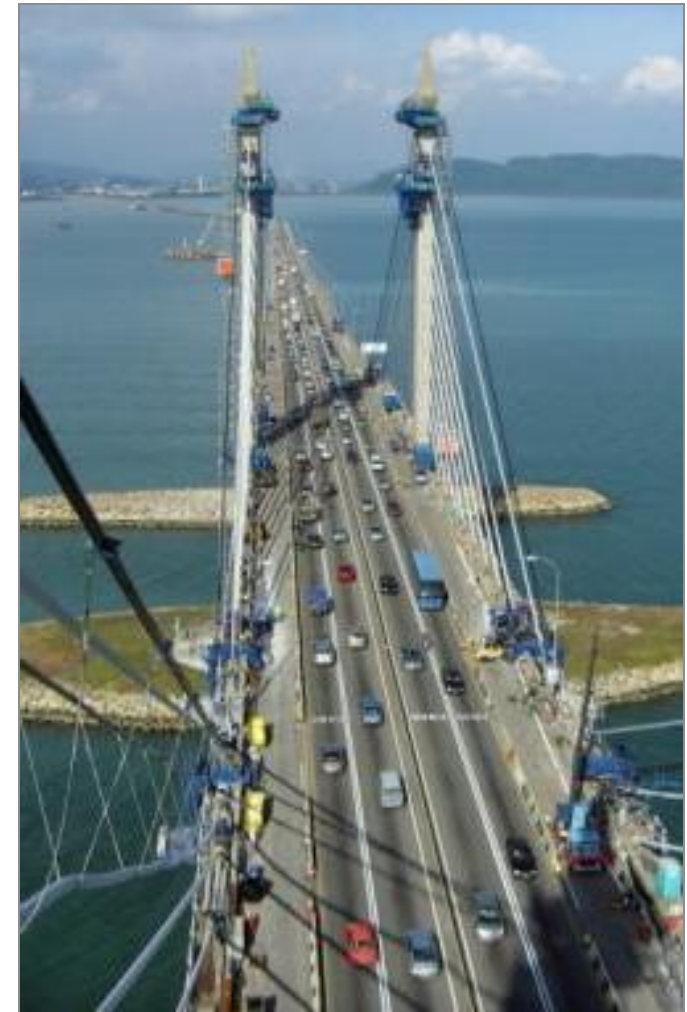
Replacing stay cables on the Penang Bridge, Malaysia
