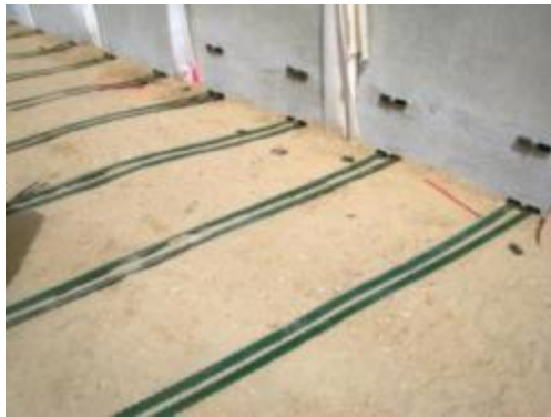
Terre Armée: “A world first for EcoStrapTM HA® reinforcements”
