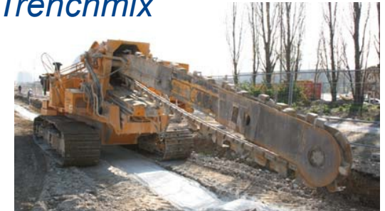
Dry method (the binder is introduced into the trench before mixing)
