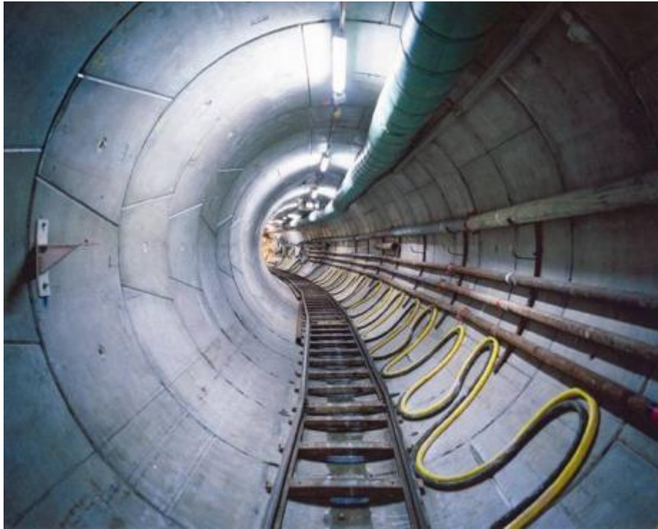
CLP Hong-Kong Tunnels for the 132 kV power cables beneath dense urban environment and under the sea
