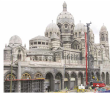
FRANCE - Marseille - Axe littoral GEOMIX retaining wall
