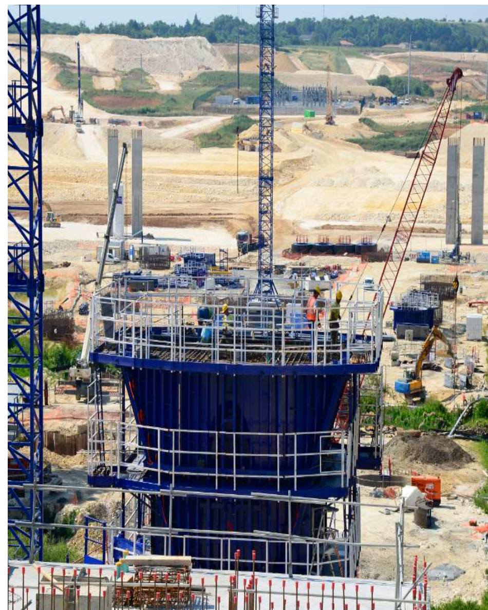
Tours-Bordeaux HSR worksite: construction of the Auxance viaducts
