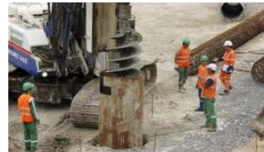
Tours-Bordeaux HSL: René Coty Bridge (Gironde)
