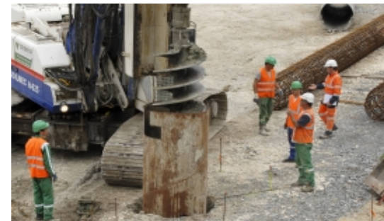
Tours-Bordeaux HSL: René Coty Bridge (Gironde)
