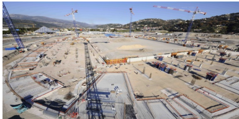
Nice stadium construction site
