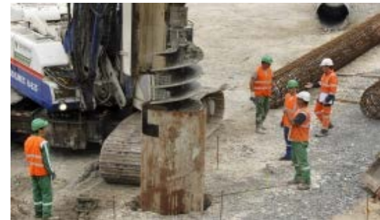
Tours-Bordeaux HSL: René Coty Bridge (Gironde)
