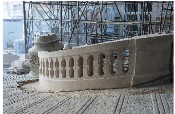
Restauration de la Cour Lefuel - Paris 1 er © Govin Sorel
