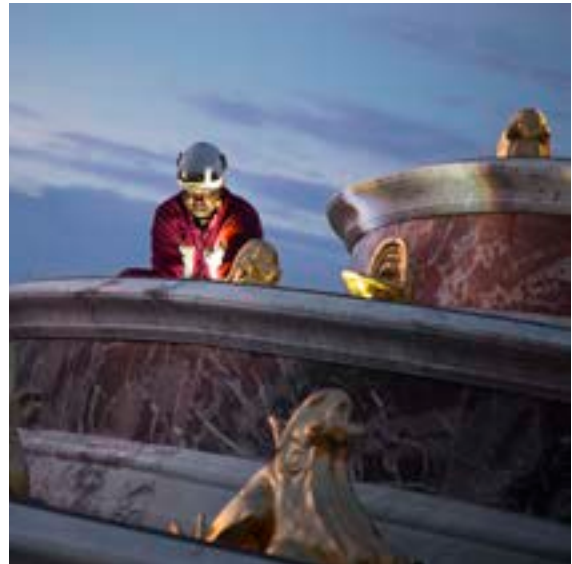
Lighting for the Latona Fountain at the Palace of Versailles.
