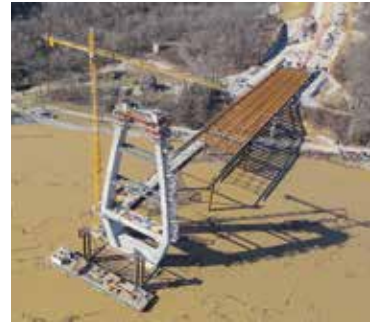
The Ohio East End Crossing project includes construction of a 762-m cable-stayed bridge crossing the Ohio River northwest of Louisville.
