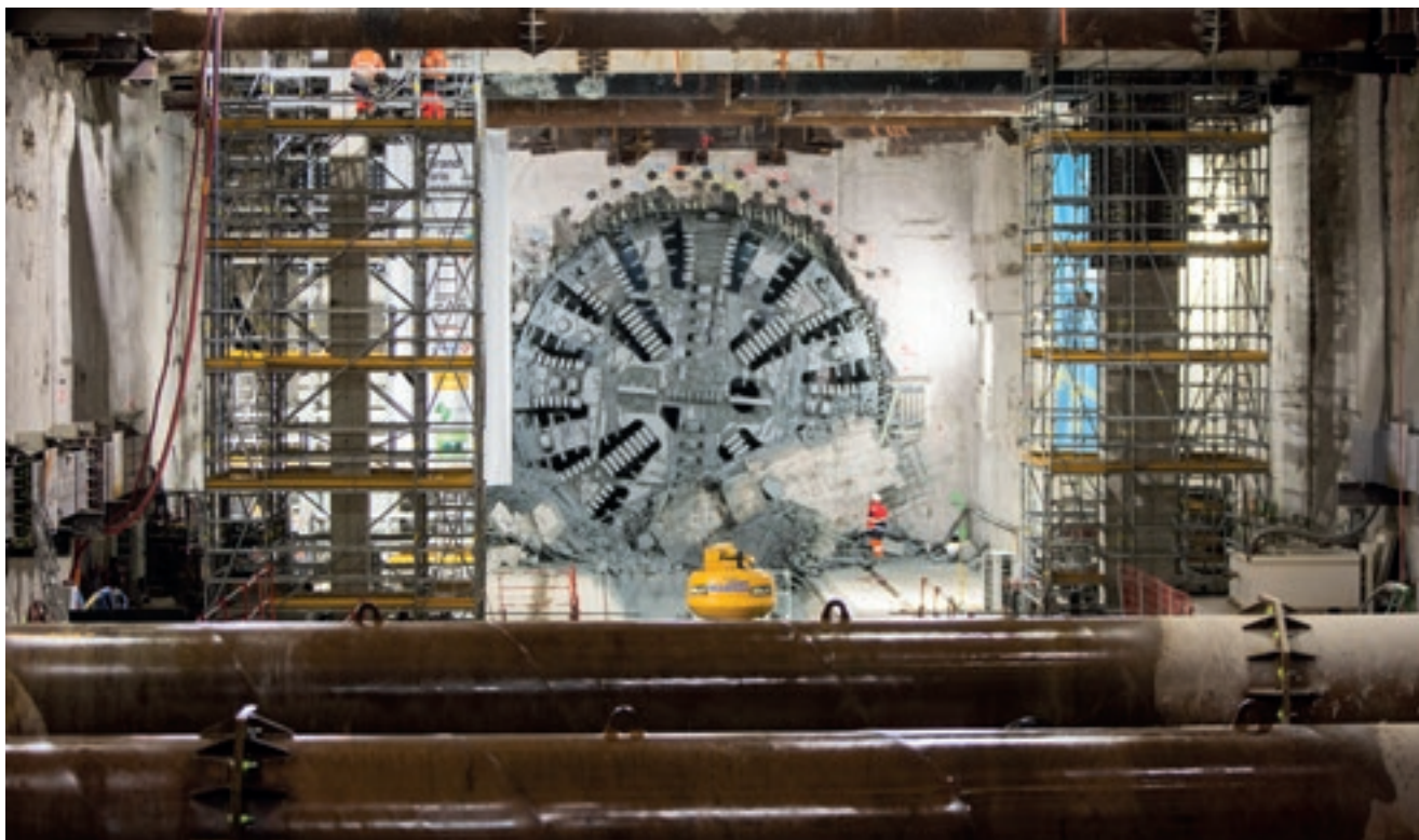
WORK ON SECTION T3C of Line 15 South of the Grand Paris Express. Tunnel-boring machine Amandine finished excavating the 3.4 km stretch between Arcueil-Cachan and Villejuif-Louis Aragon stations.
