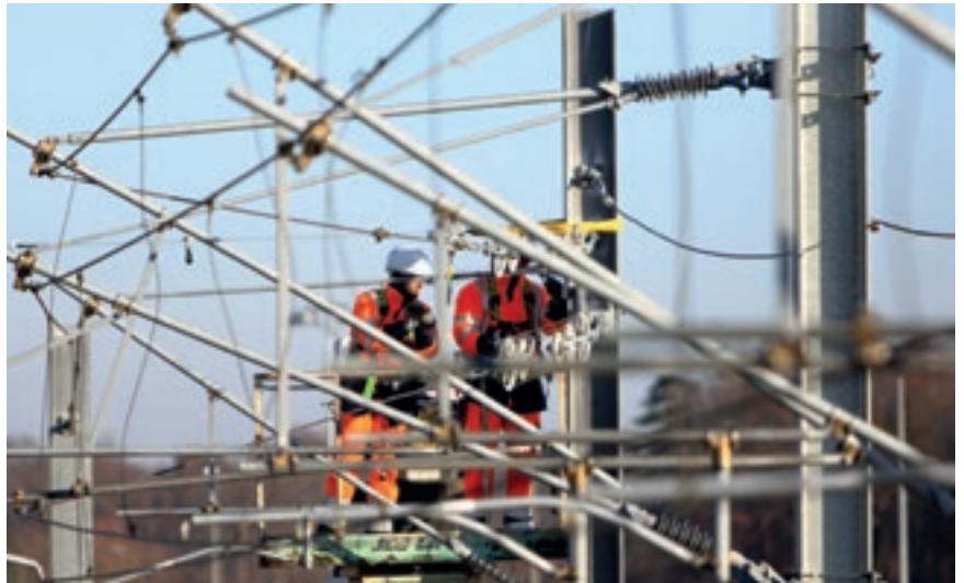
MAINTENANCE of the electric power infrastructure for trains on the SEA HSL Tours-Bordeaux.
