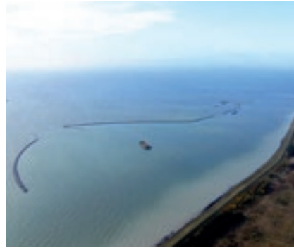
DENMARK Work begins on the Fehmarnbelt Fixed Link, the world's longest immersed road and rail tunnel (17.6 km) between Denmark and Germany.
