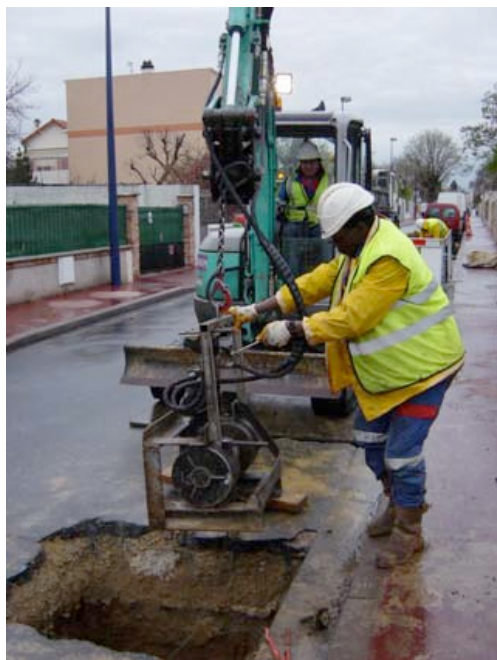
Replacement of 4,000 lead service pipes in 16 districts to the south-west of Paris
