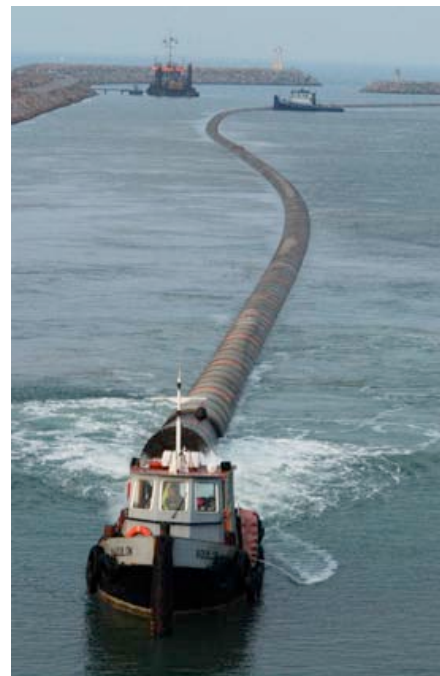
The 11 km sea outfall for the Montpellier wastewater treatment plant
