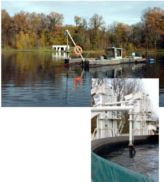
Dredging operation in the lake at Vélizy and extraction at sludge plant
