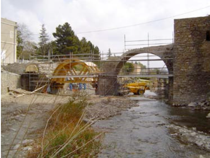
Installation of scaffold on the Cascatel des Corbières bridge to carry out diagnostics
